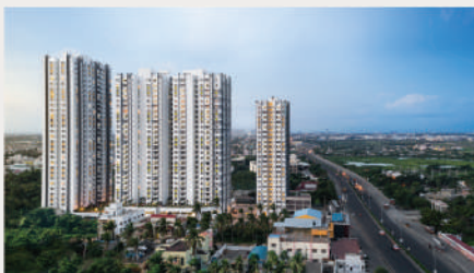
Tallest Residential Skyscraper within Chennai Limits, Sholinganallur, OMR.
